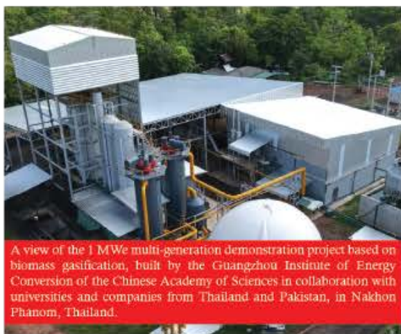
A view of the 1 MWe multi-generation demonstration project based on biomass gasification, built by the Guangzhou Institute of Energy Conversion of the Chinese Academy of Sciences in collaboration with universities and companies from Thailand and Pakistan, in Nakhon Phanom, Thailand.
